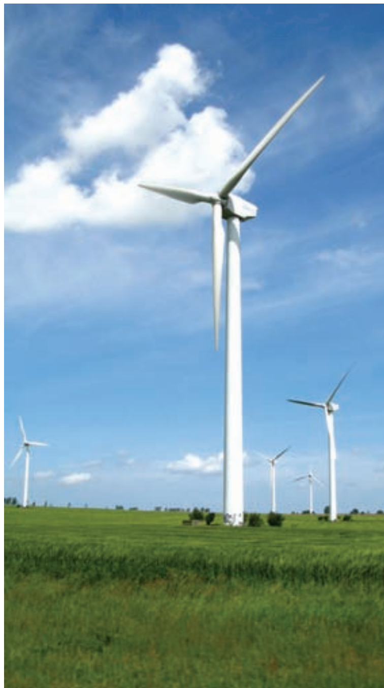
Locals blowing hot air: Resident reaction has been mixed during the consultation process despite the university radically improving its green credentials with the two new turbines
